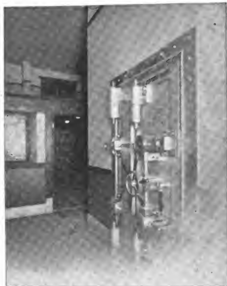
Safety Deposit Vault.
